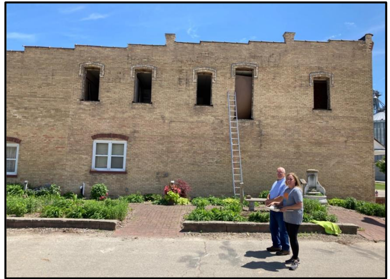
Windows were removed and bricked up courtesy of Schuh Construction and Pahlow Masonry.
