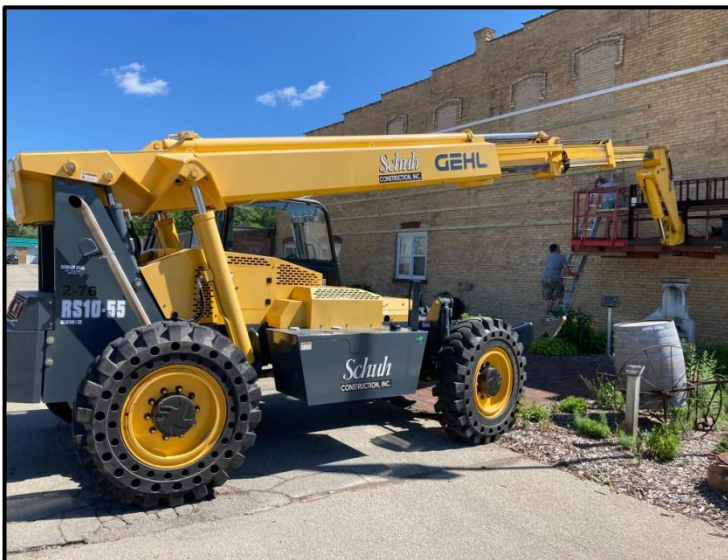
Schuh Construction installed a base to which the aluminum panels were attached.
