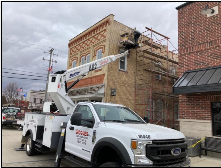
The former Miller-Piehl office building (1893) was cleaned and worn bricks and mortar were replaced.
